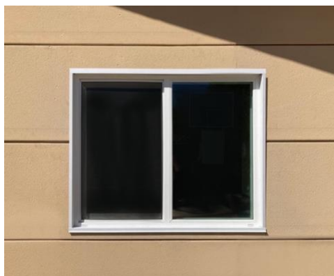
Figure 18. Use aluminum window closures.
